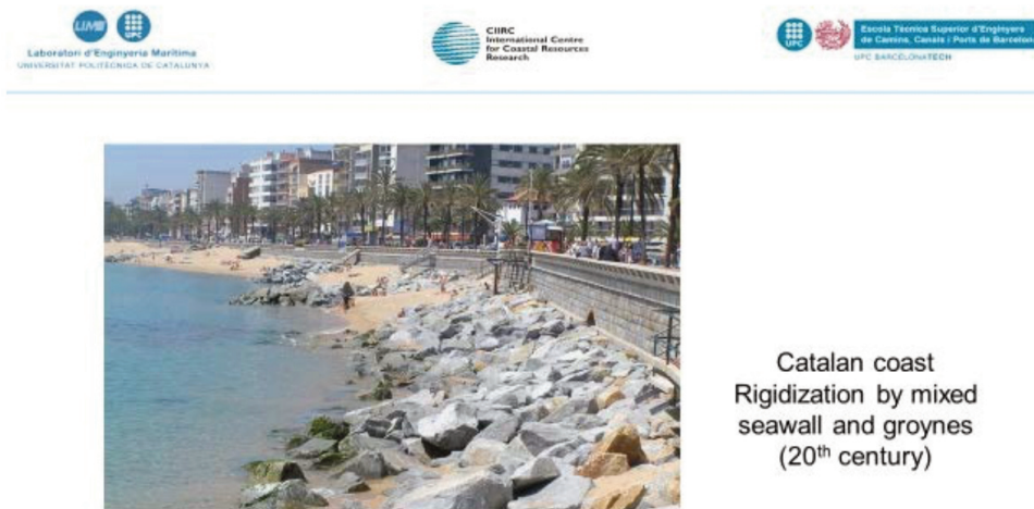
Figure 4: Illustration of rigid coastal protection by groynes and alongshore revetment for a stretch of heavily urbanised coast in the Spanish Mediterranean
